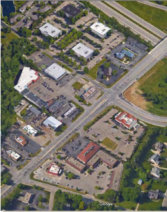
FIGURE 20: EXAMPLE OF INTERSTATE HIGHWAY
